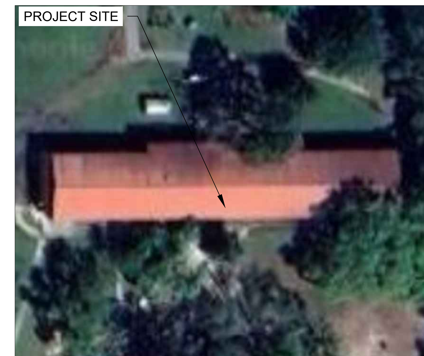
1 BUILDING PHOTO SCALE: NTS
